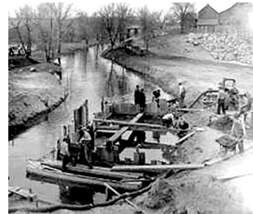
Waterworks canal to Saint Paul connecting Lake Vadnais to Sucker Lake. Image 1937 MNHS
