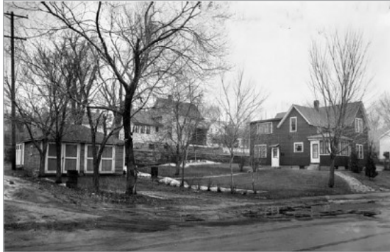
1213 Pleasant was built in 1903 for Mrs. M M Hohmann and removed in 1967 for 35E. Image 1956 RCHS
